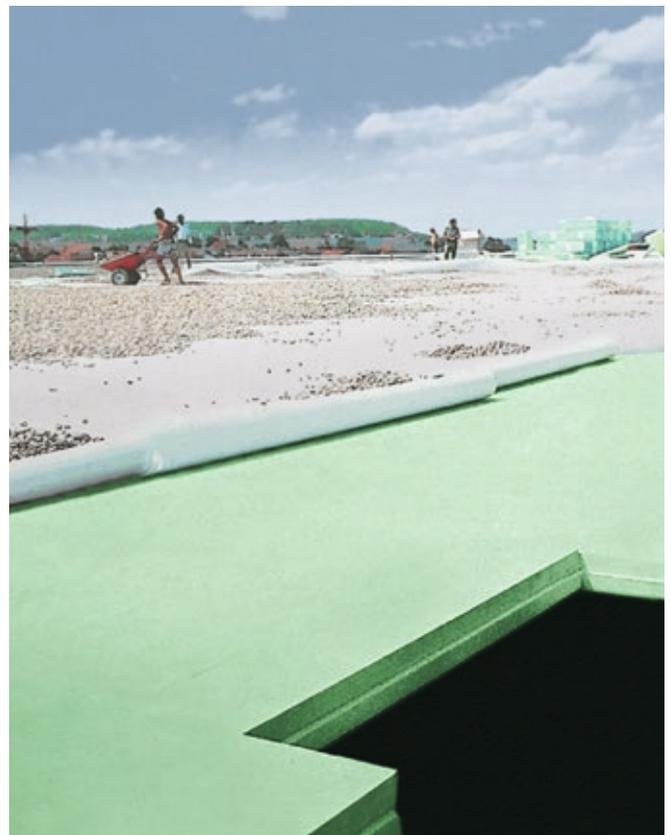
**Fig. 9:** Inverted roof with separation layer and gravel.
