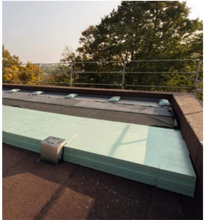
**Fig. 1:** Thanks to its compressive strength, low water absorption, and low thermal conductivity, Styrodur® is perfectly suited for inverted roof structures, such as plus roofs for flat roof renovations.
