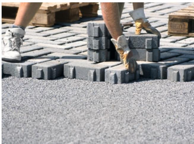
**Fig. 45:** Composite stone pavement with grass joints for a parking roof on top of a gymnasium.
