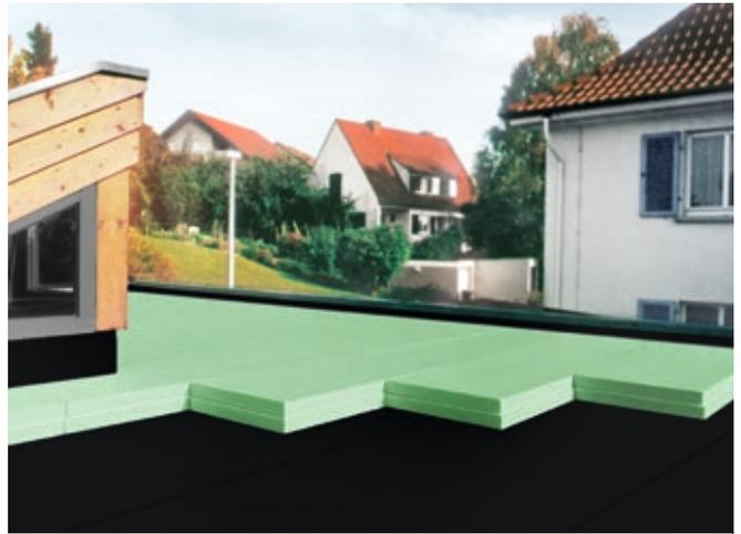
Fig. 25: Installation of Styrodur® boards under an extensive green roof.
