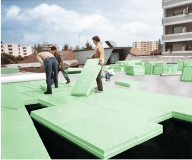
**Fig. 12:** Installation of Styrodur® for a duo roof.
