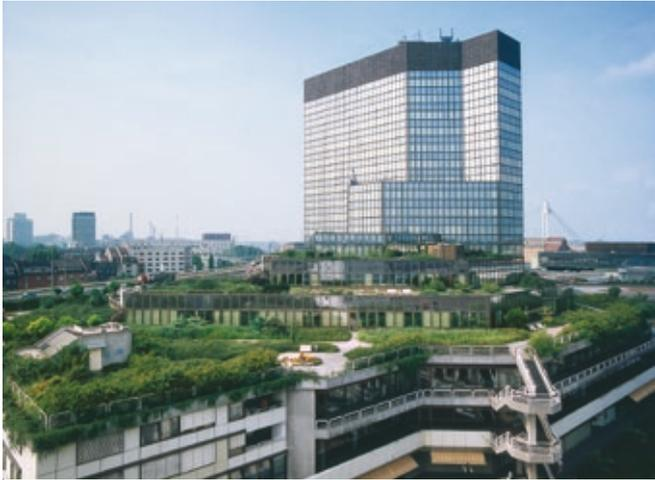
**Fig. 27:** Intensive green inverted roof.
