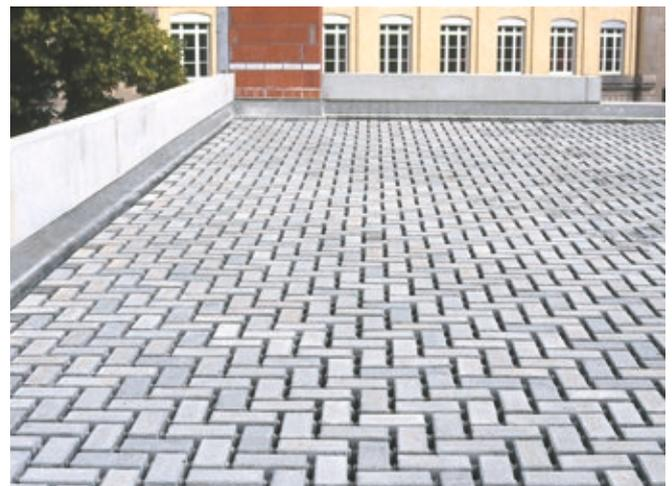
**Fig. 47:** Concrete pavement on Styrodur® boards.
