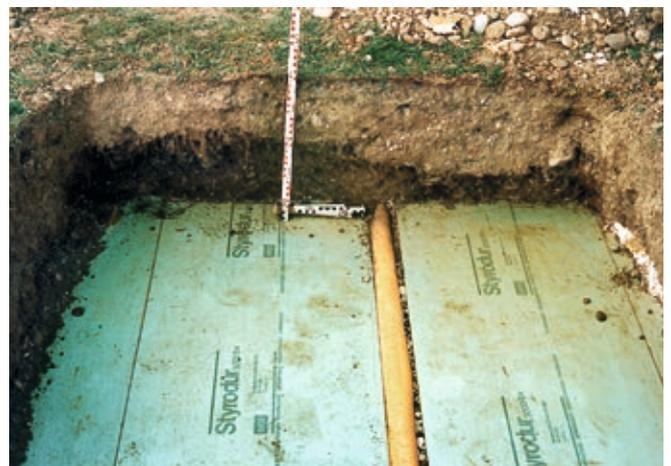
**Fig. 6:** Image shows a green inverted roof that is more than 30 years old
