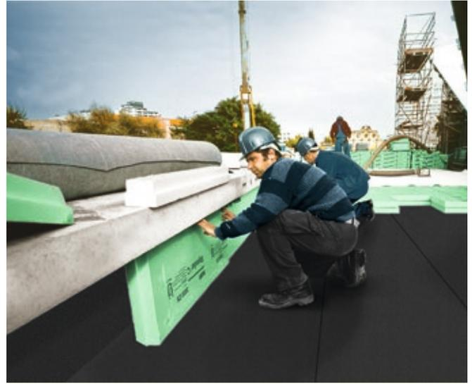
**Fig. 13:** Parapet insulation with Styrodur®.
