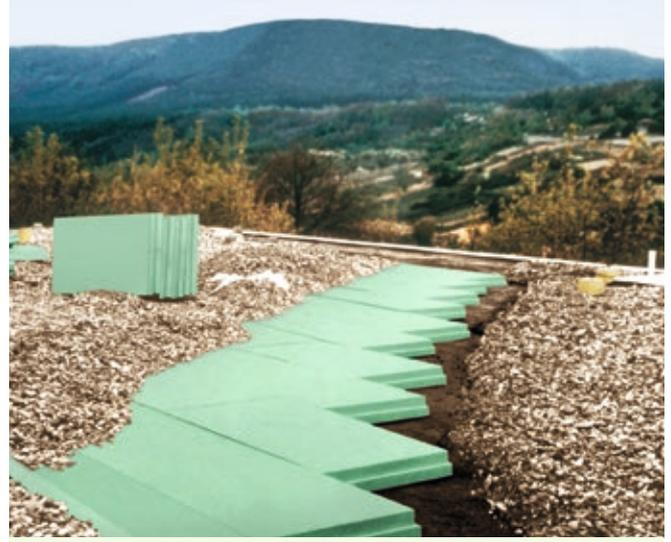
**Fig. 16:** Renovated inverted roof as a plus roof.
