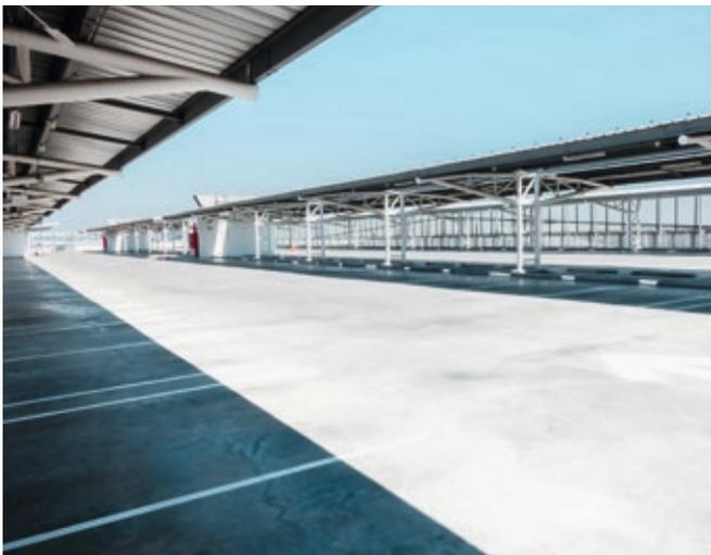
**Fig. 49:** Parking roof with in-situ concrete driving surface.
