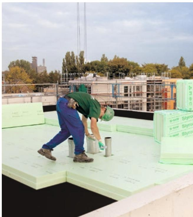
Fig. 3: Inverted roof insulation with Styrodur® for 250 housing units in Hamburg.
