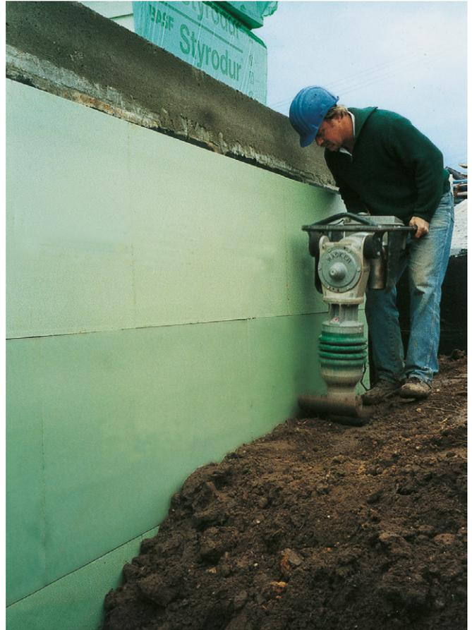
Fig. 18: Layered backfilling of the excavation pit and mechanical compacting
