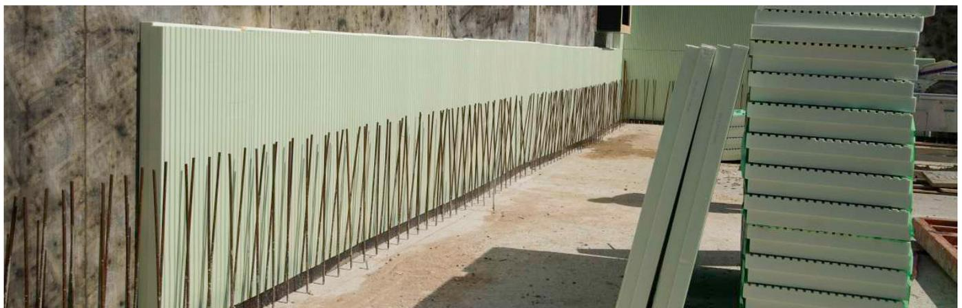
Fig. 4: Installation of Styrodur Hybrid on the inside of the formwork.
