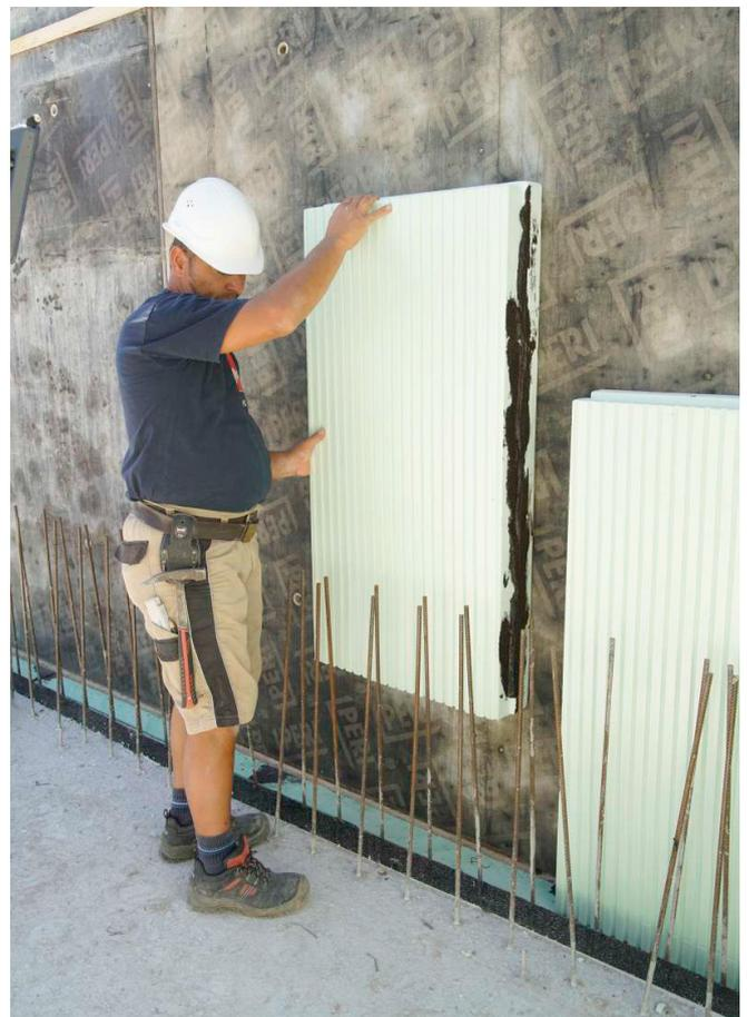
**Fig. 7:** Positioning the Styrodur Hybrid boards.
