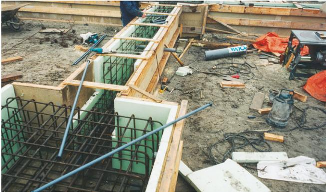
Fig. 16: Formwork with Styrodur Hybrid.
