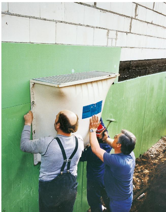
Fig. 13: Fitting a lightwell.
