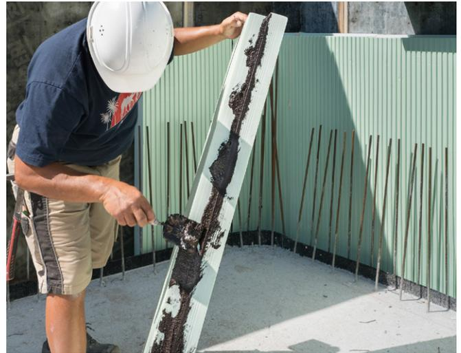
**Fig. 6:** Sealing the board edges against pressing water.
